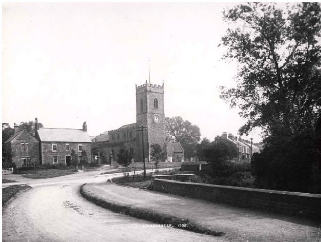
Before and after the by pass
